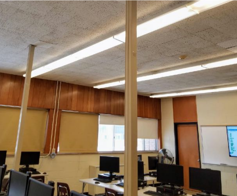
Fluorescent Lights and Poorly Insulated Ceiling Enclosure
