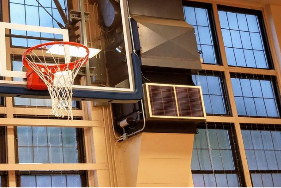
1960's Vintage Air Handling Unit and Poorly Insulated Windows
