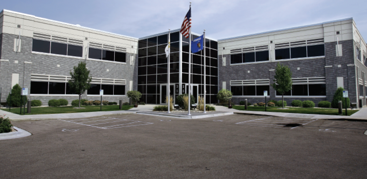
T.E.C. Incubator Center is located near MATC's Truax Campus, which often supplies trained technical workers.
